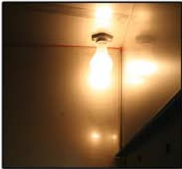
2 interior lights with teflon coating prevent shattering.
