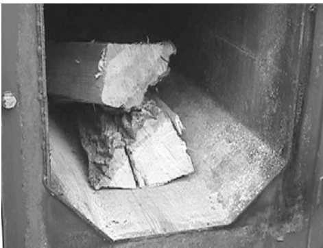
Correct way to load wood. Use 1, 2 or 3 hardwood logs, 4-6 inches in diameter, 12-15 inches long.
